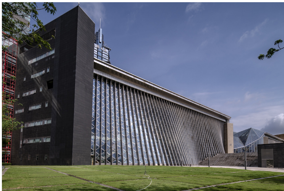
Figure 3. The exterior facade of the Shenzhen Library.
