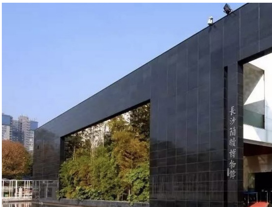
Figure 2. The exterior façade of the Changsha Bamboo Slips Museum.
